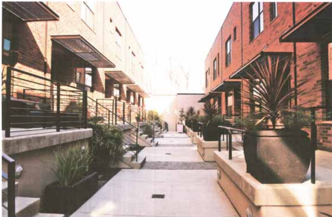
The homes at Sutter Brownstones open onto two courtyards separated from the street with a short flight of steps. The patios give the project a sense of community, but the detached homes offer some privacy as well. The judges liked the project's "natural separation" from the sidewalk.
