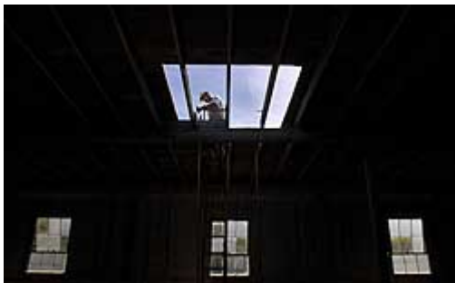
Louis Lentine works on an elevator shaft above what will be a third-floor art gallery in the Paragary project.
